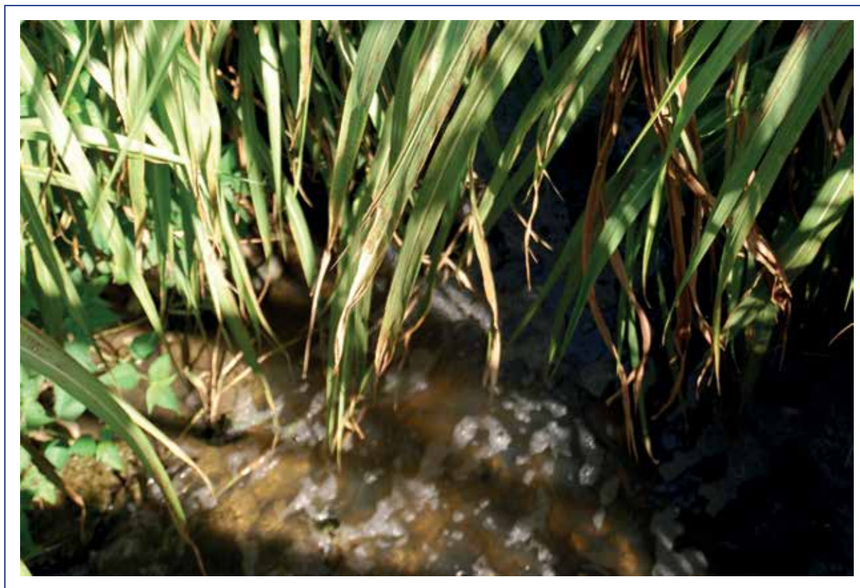
Figure 5.11 Nutrient rich effluent from the Knysna Waste Water Treatment Plant entering a reed bed prior to discharge into the estuary (Photograph: © Alan Whitfield).
